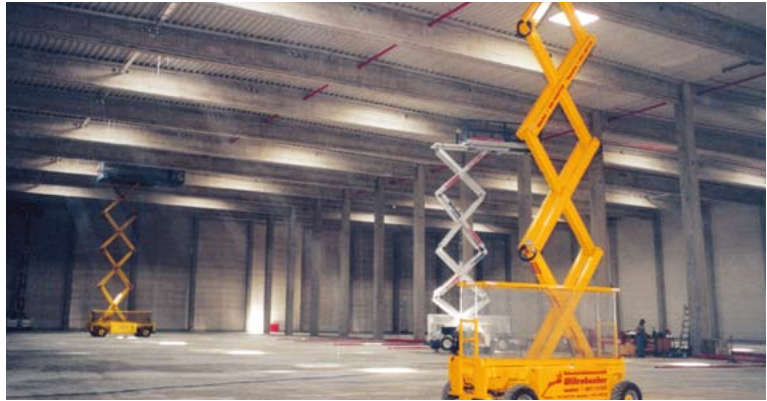
TNT logistics centre in Niederaichbach with Düker SML cast iron drainage pipes.
